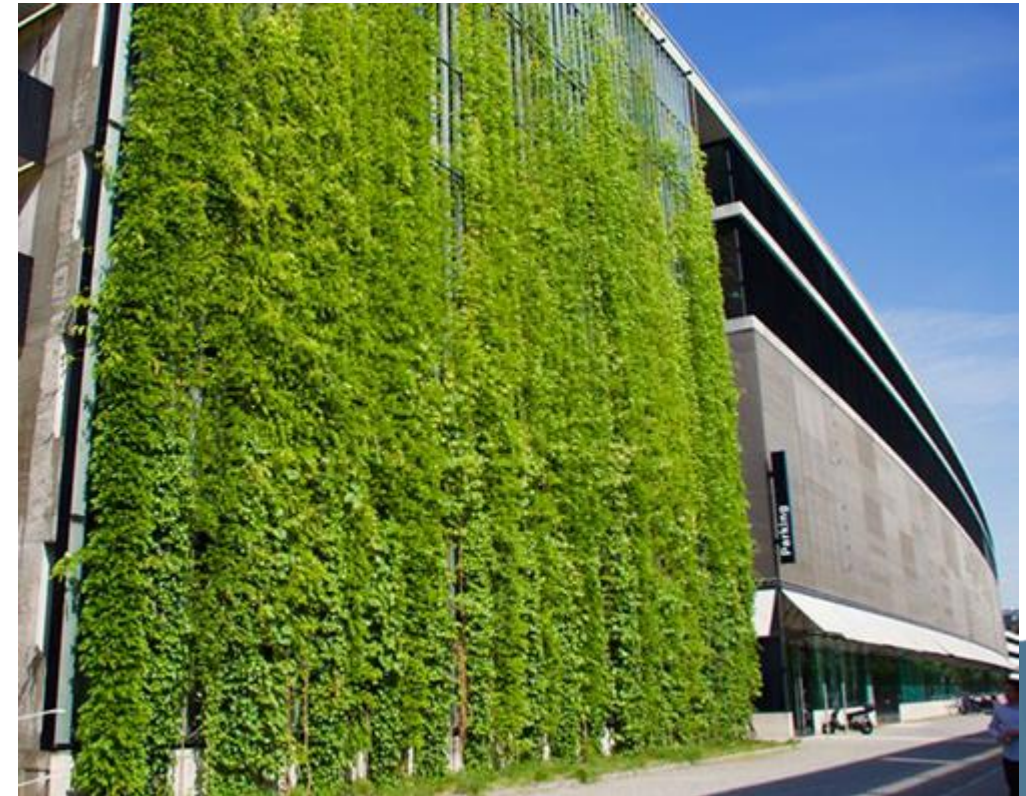
Source: LivingRoofs.org A cable-supported vertical green wall installed on the facade of a building in Switzerland.
