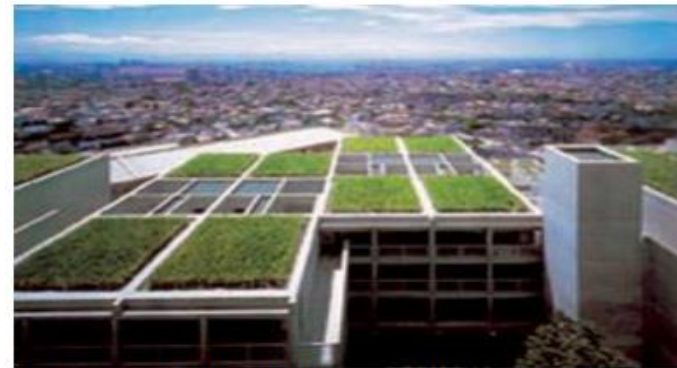
Examples of Extensive Green Roofs
